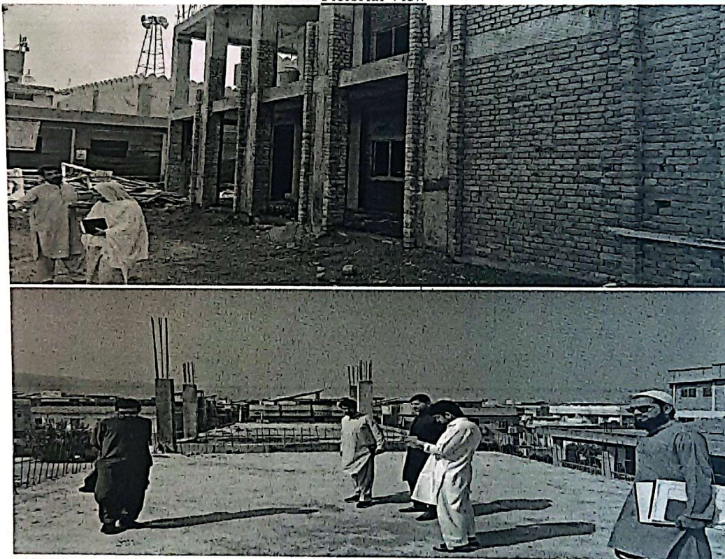
Inspection Committee site visit GPS No 3 Hayatabad: 4 ACR and P2M
